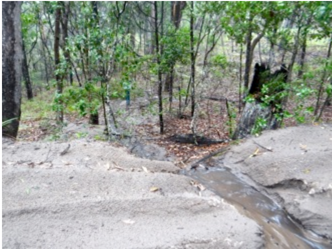
Sediment moving from road to Coolooli Monitor site
