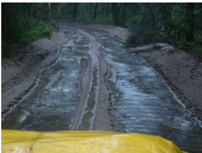
The road in was a raging torrent
