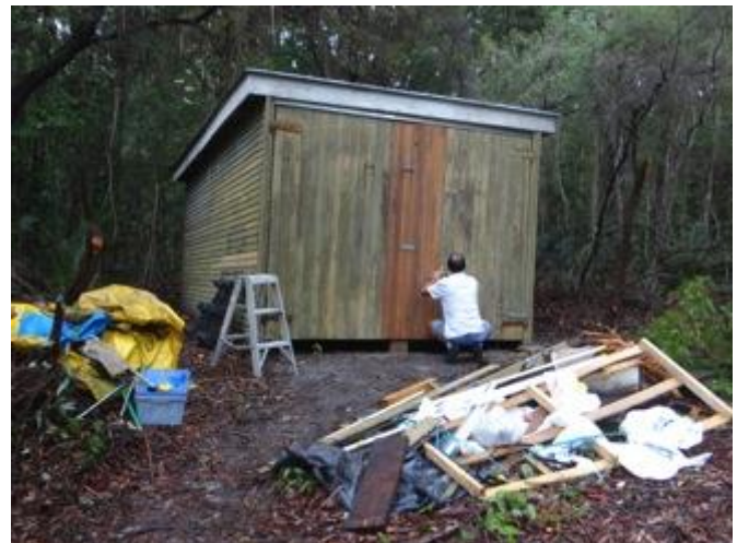
Neville works on the doors of the storage shed that was almost overgrown before our arrival
