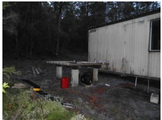
The tank-stand had a new deck made up with sleepers that formerly flanked Lake McKenzie (Boorangoora)'s shores. When the 5 tonnes of water were added one post wouldn't carry the full load and subsided a little
