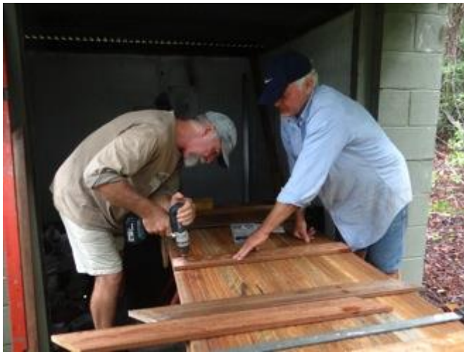
Noel and Eric using up the last of the power to complete the doors to secure the Generator shed
