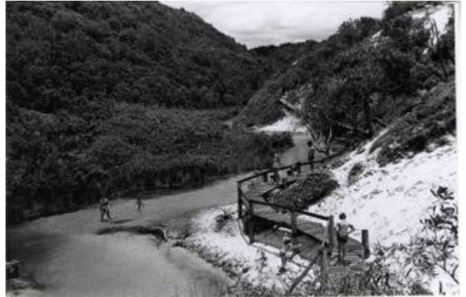
The completed boardwalk enabled the creek-side vegetation to re-establish and the creek soon deepened. FIDO did a lot of planting to help the healing. The scarring quickly overgrew.
