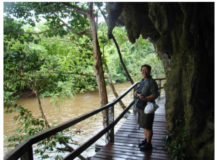
This is one of the boardwalks constructed between the most popular destinations in the park so that few of the 35,000 visitors ever leave a hardened path during their visit to Mulu Park.
