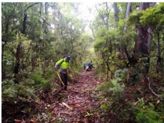
The standard for track clearing adopted was that the track should be obstacle cleared for walkers but wide enough to allow the passage of a small tractor for future maintenance where the tracks are using former roads.
