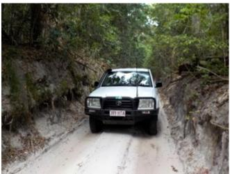
This 2 metre deep gash on the Woralie track extends for 300 metres. It has been eroded by rain and is so deep that one can't see the surrounding rainforest. It developed in less than 40 years.
