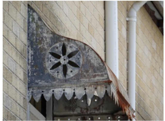
Some of the most decrepit and neglected older homes of Maryborough had gems of creative vernacular architecture, such as this use of galvanized iron.
